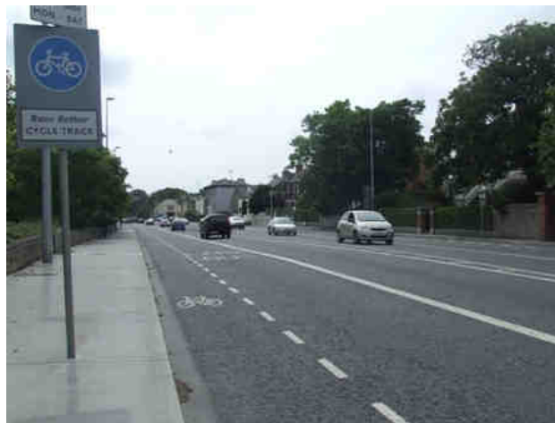
Existing cycle lane and bus lane – insufficient widths
