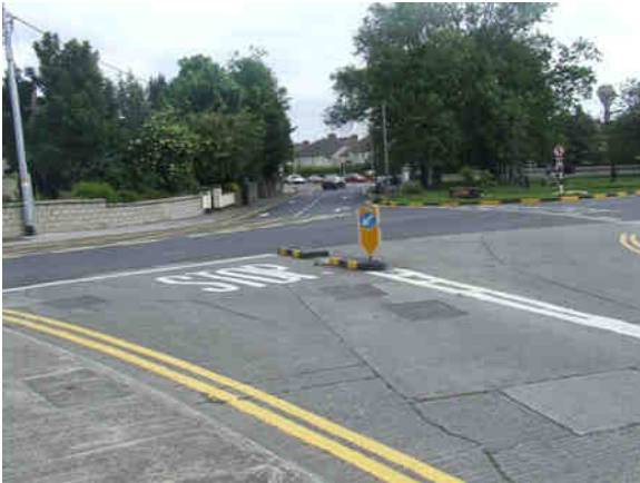
Gledswood Park – Bird Avenue, kerb build out to improve crossing for pedestrians and cyclists
