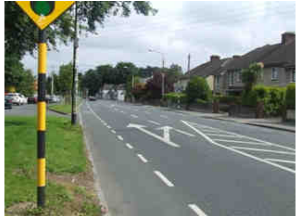
Existing cycle lanes (1.2m) on Clonskeagh Rd to be widened to 2m
