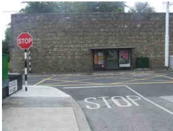
Exit at St Columbanus Road, cyclist will ramp up here to proposed shared space
