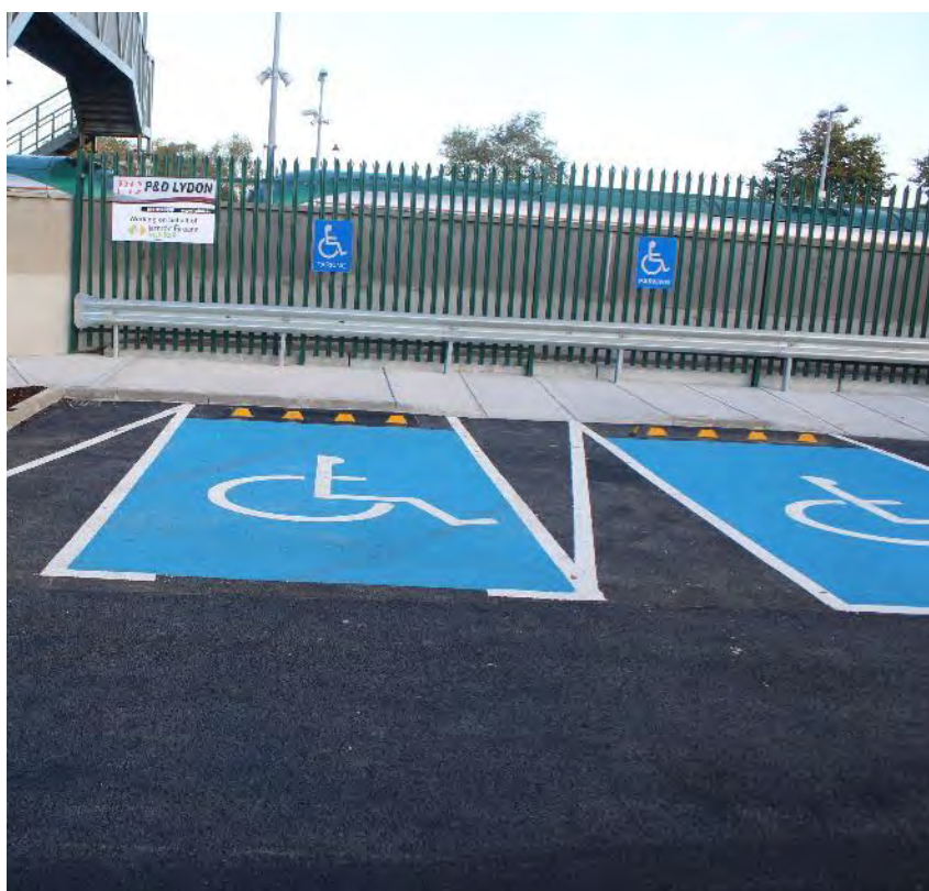
Figure 1 Example of recently constructed PRM parking at Maynooth station
