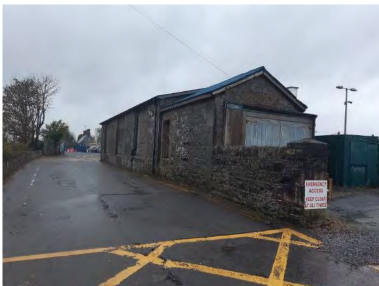
Figure 77 Existing Permanent Way building (looking North East)
